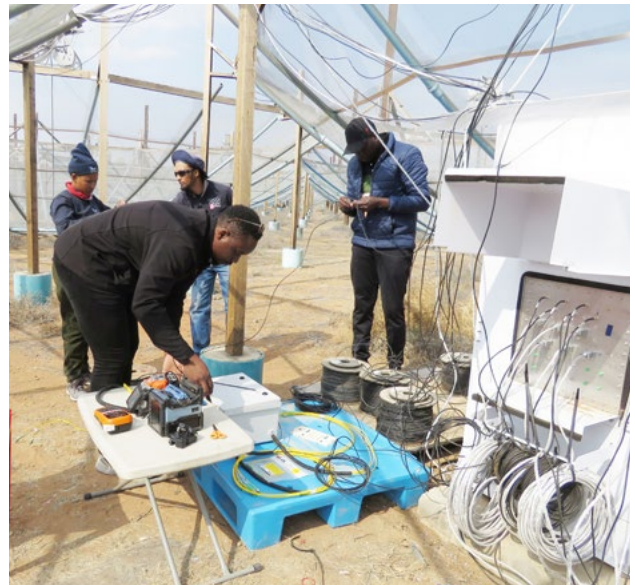
Dr James Jena (postdoc) and Dr Victor Agbakoba (postdoc) preparing to install the delay lines to HERA telescopes
